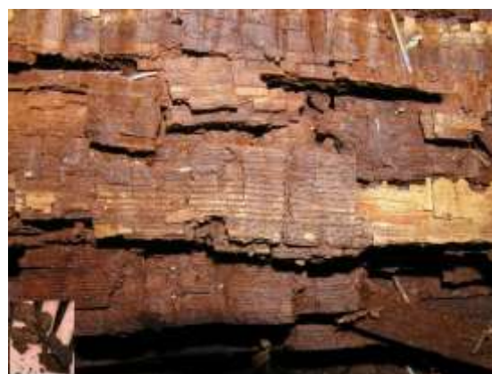
Figure 3: Rotten timber, as shown above, will weaken the structure and attached mesh leaving rabbits vulnerable to attack. (photo credit: Beentree)
